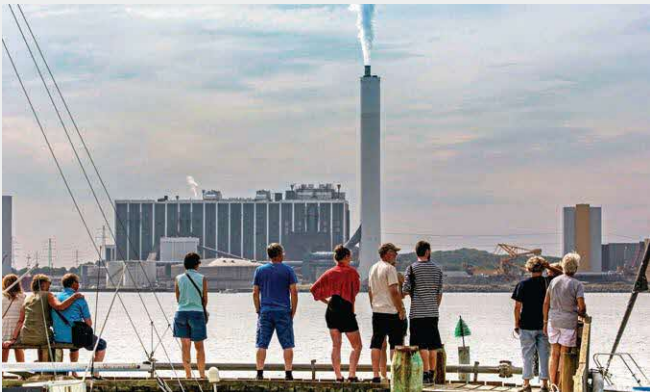
The Asnæs Power Plant forms a key part of the Kalundborg Symbiosis. By-products and waste from the power plant are used by other manufacturers in their own production lines. Photos courtesy of (top) Johan Wessman / News Øresund (CC BY-SA 2.0 / Wikimedia Commons) and (bottom) Bob Collowan (CC BY-SA 3.0 / Wikimedia Commons)
