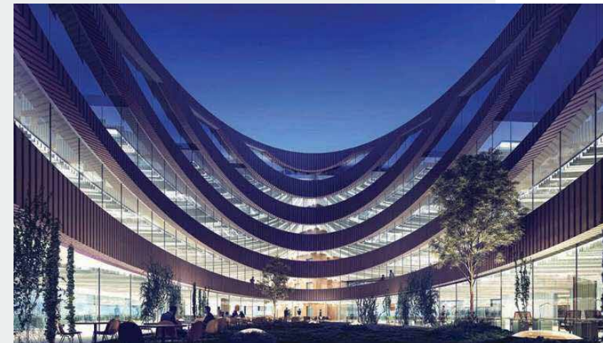
A view of the building's atrium and public garden; the space was designed to optimise daylighting and natural ventilation.
