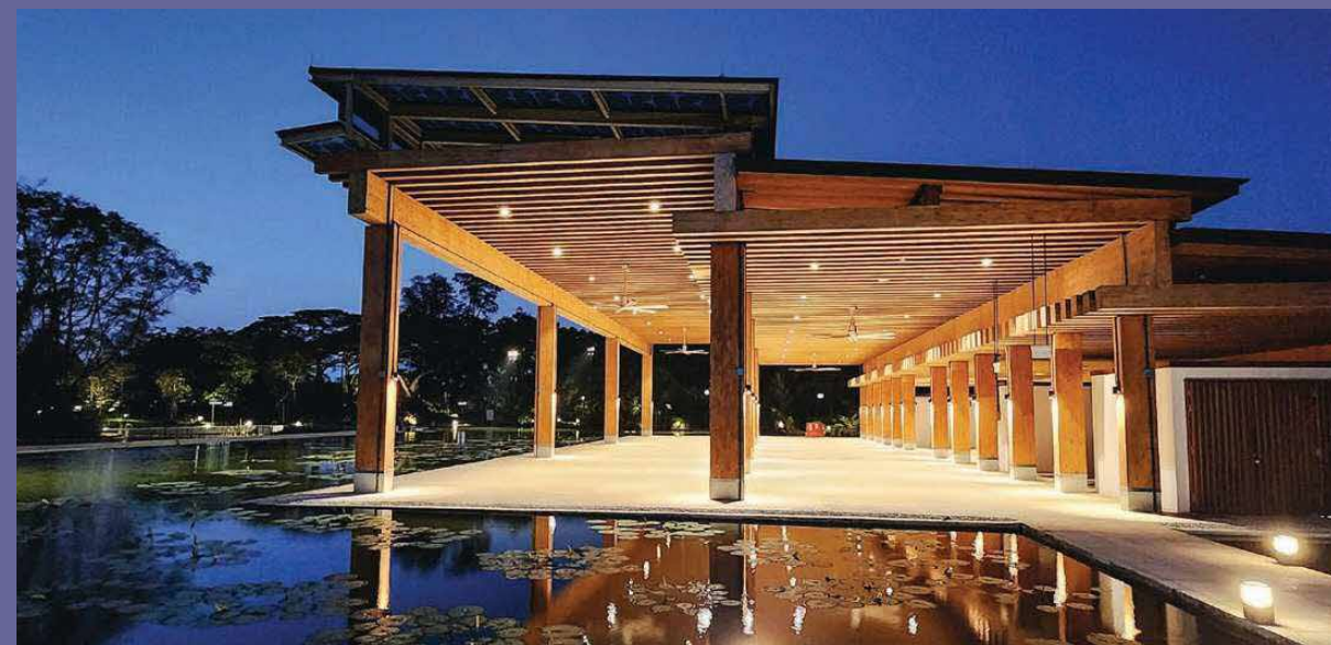
At Jurong Lake Garden's Japanese Garden, advanced Mass Engineered Timber was used as a sustainable innovation for construction of the Water Lily Pavilion (above) and the Guesthouse (left).
