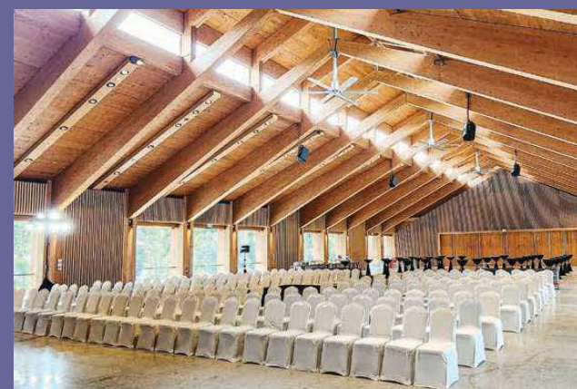
At Jurong Lake Garden's Japanese Garden, advanced Mass Engineered Timber was used as a sustainable innovation for construction of the Water Lily Pavilion (above) and the Guesthouse (left).
