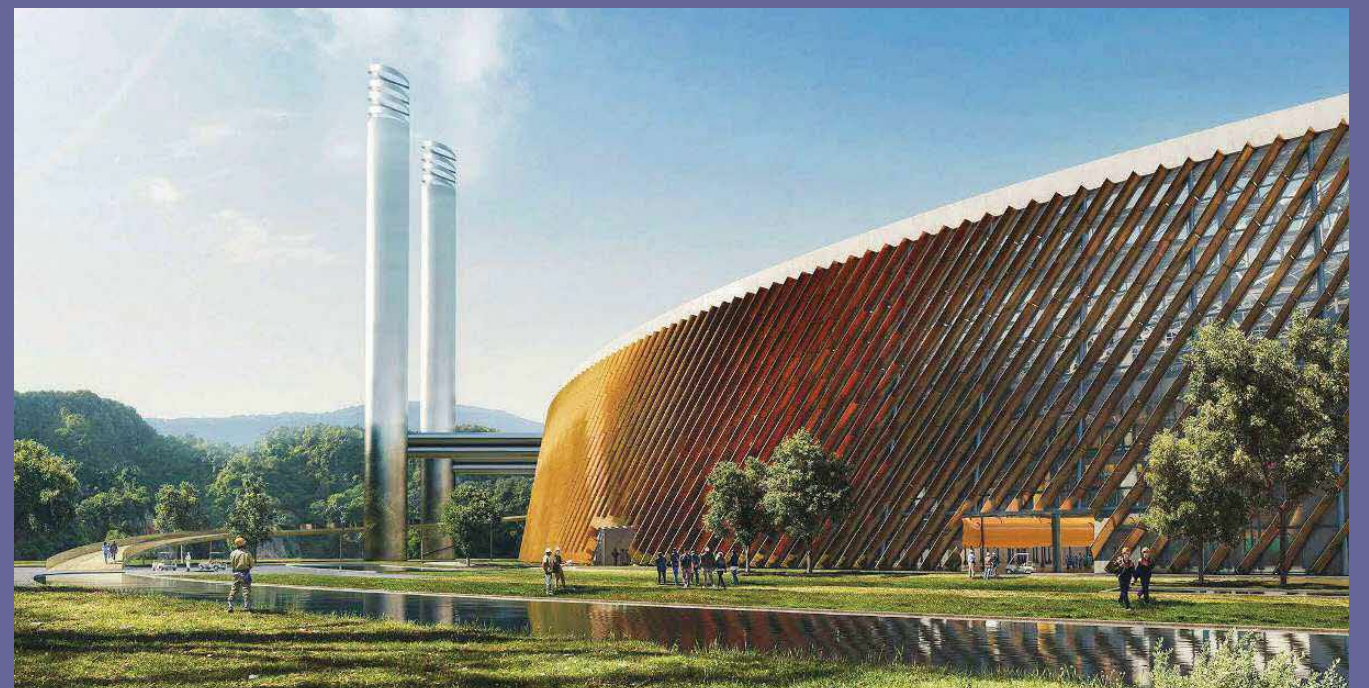
Shenzhen advances a low-carbon transition through coordinated urban systems—integrating emissions reduction into everyday operations while strengthening resilience and circular infrastructure—at the Huaqiangbei Ganquan Road Near-Zero Carbon Community (top) and other industrial parks and public facilities (bottom). Photo and image courtesy of Shenzhen Urban Planning and Land Resource Research Center
