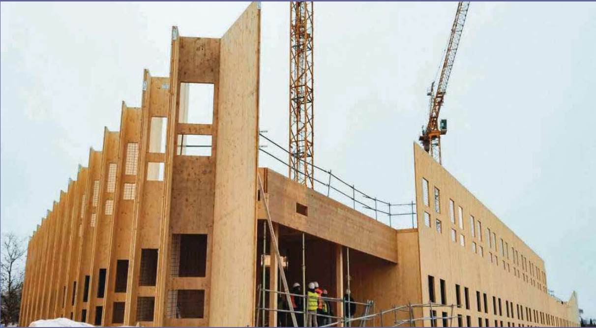
The Campus for Living Cities in the South Campus of Madrid’s Polytechnic University was set to be Spain’s largest cross-laminated timber building in 2025. Photo courtesy of ©UNEXUM
